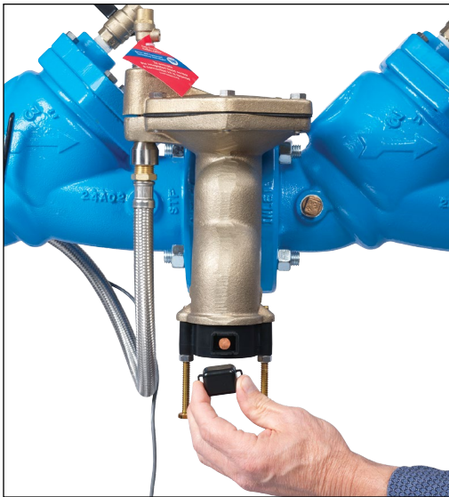
1. Remove the dust cover from the sensor.
